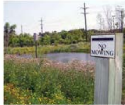
Detention basin with a no mow buffer in West Bloomfield Township, MI Source: Hubbell, Roth, & Clark
